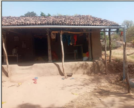
Roof top harvesting system for open well recharge
