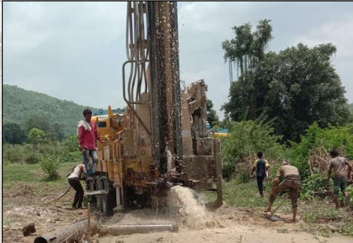
Drilling of Bore well
